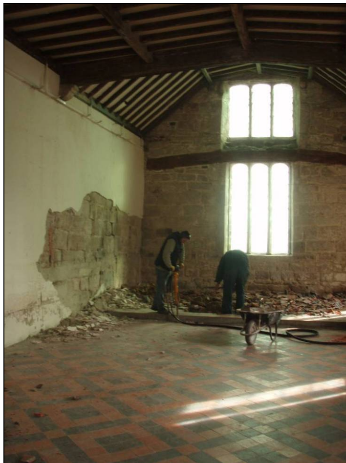
Figure 19 Work to remove the Victorian floor level.
