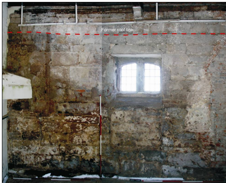
Figure 6 Window opening at the western end of the north wall with lower section blocked up. (Scale: 2m)
