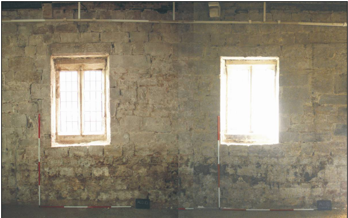
Figure 8 The two later windows within the southern wall. (Scale: 2m)
