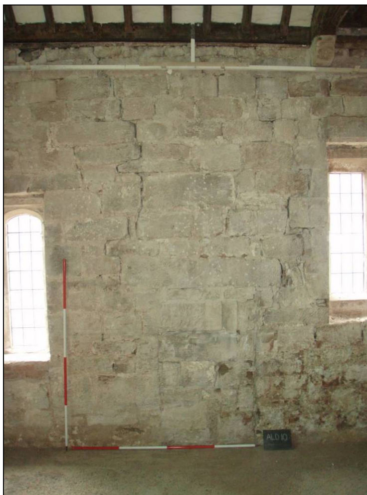
Figure 11 Blocked doorway in the south wall. (Scale: 2m)
