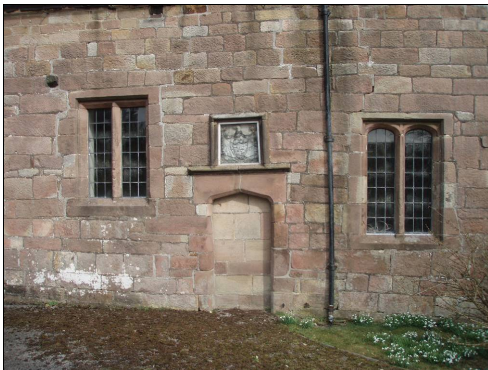
Figure 9 Exterior of south wall showing height difference between the windows and the lower sloping quadrilateral shaped lower courses.
