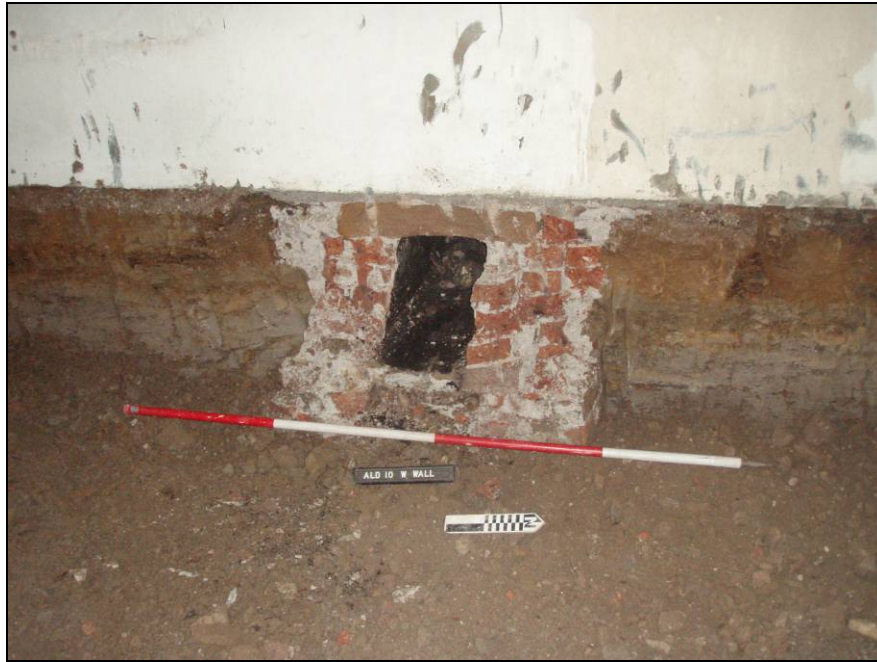
Figure 16 Victorian drain located within western elevation below modern ground level. (Scale: 2m)
