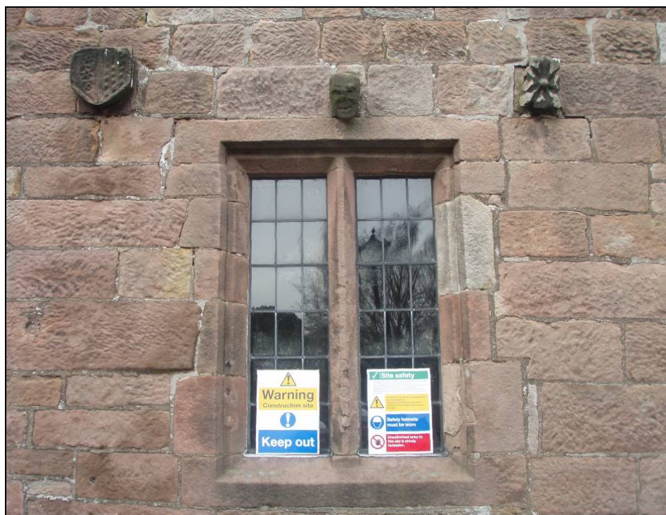
Figure 10 Exterior of south wall showing inserts around the later windows.
