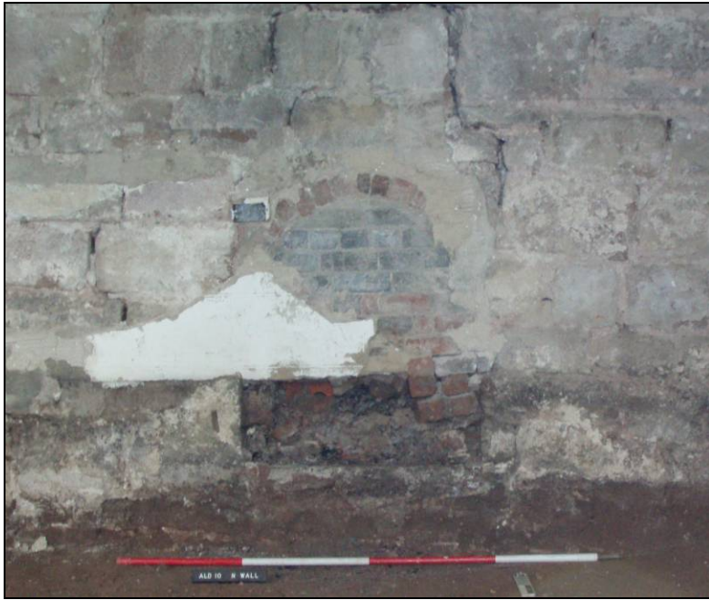
Figure 4 Inserted brick fireplace in north wall following the removal of flooring. (Scale: 2m)
